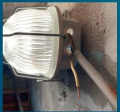
With a twinkle in his eye, he writes: "I now know why a ship fitting like this has two cable entries. Actually, a third cable entry is missing. Then you could also feed the PE into the light as well, even if it is not actually required."
