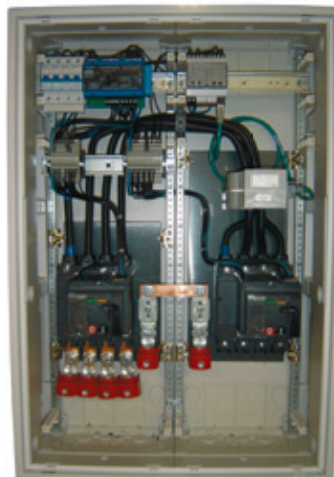
Structure of grid and plant protection with additional integrated fire safety via DMRC 1B+, DCT 70B+ and DTCC-1 (left: Gustav Hensel GmbH & Co. KG, right: ABN Braun AG)
